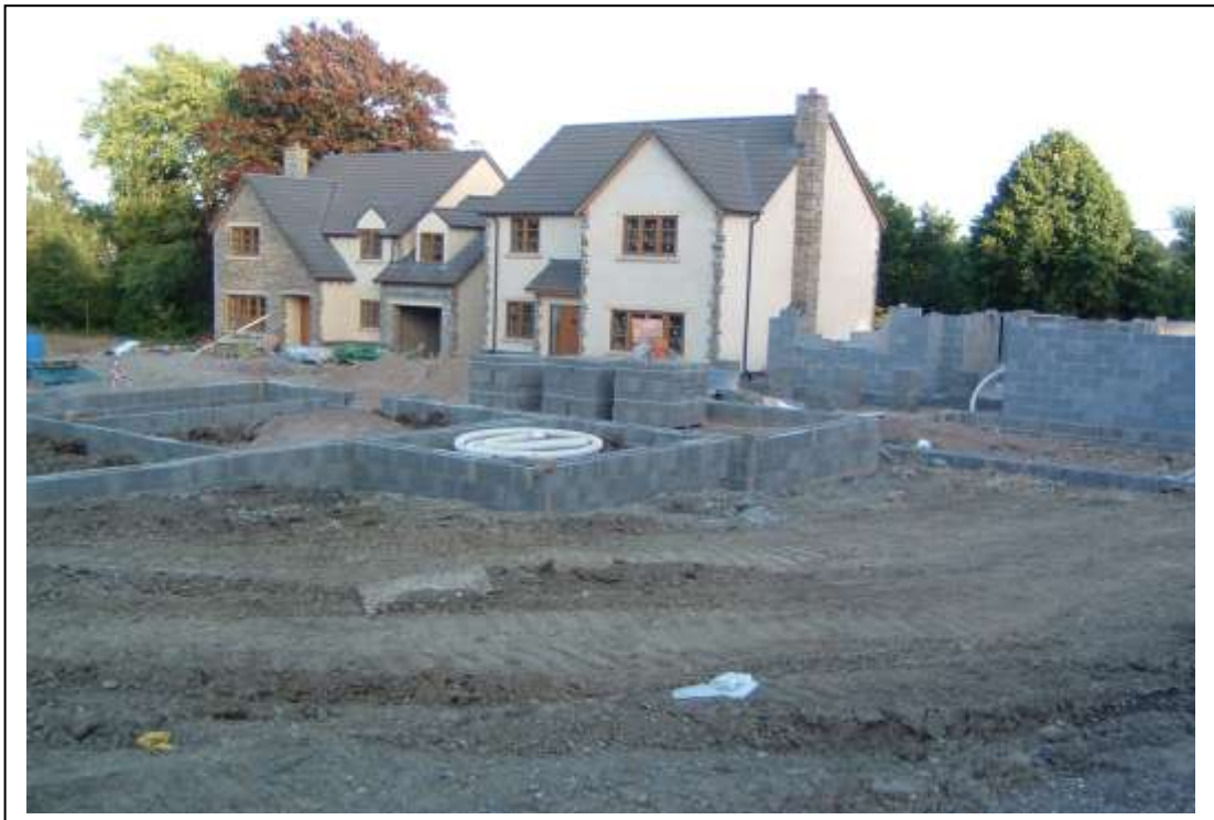
Housing Development at The Sidings under construction
