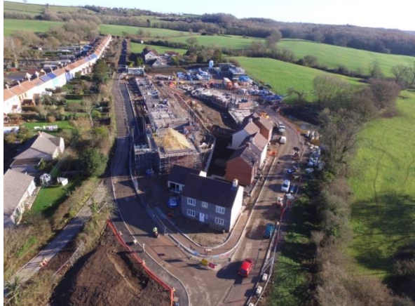
Above: Aerial shot of construction works at Highbury Fields (January 2019)
