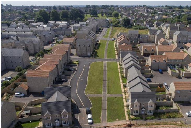
Above: Aerial image of High View, Paulton
