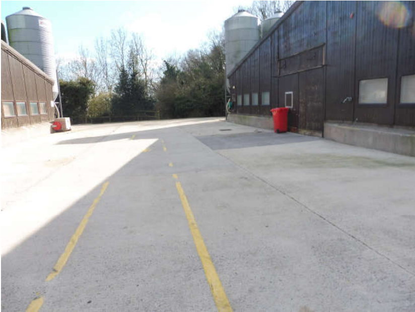
Figure 2.4 Existing FP over flight of steps between Poultry Houses.
