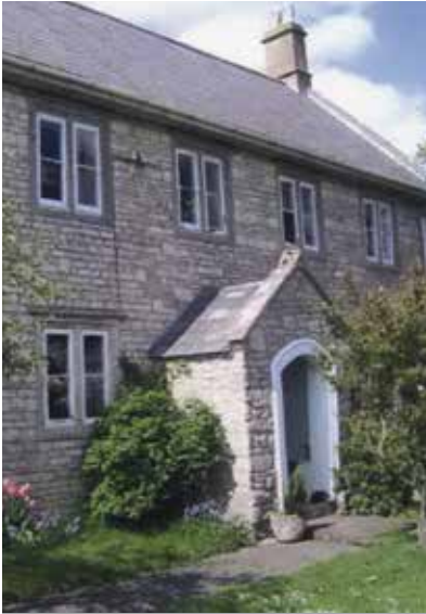
B) New slim-profile double-glazed units in Grade II listed building (Tunley Farmhouse, Tunley Hill, Camerton; view application)
