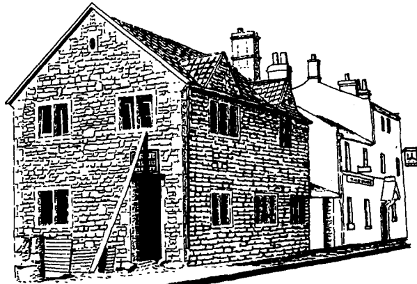
Fig: 14. Reconstruction of cottage using reclaimed oolitic limestone - an example of good craftsmanship with stone correctly "laid on bed".
