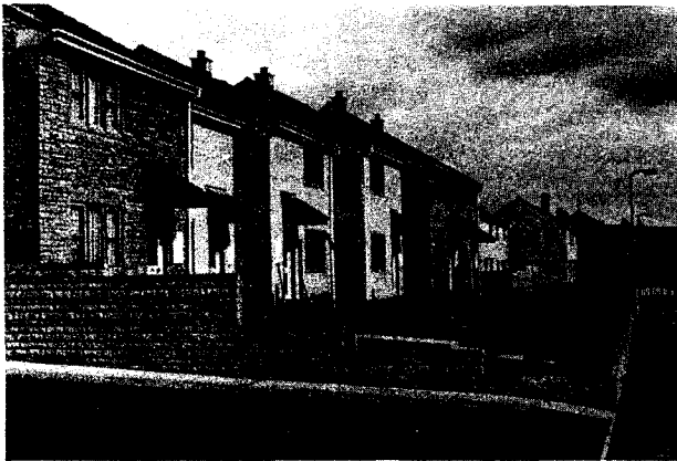
Fig: 7. Reconstructed stone of the correct colour and texture can be successfully mixed with cement and sand render. Local authority housing at Welton).
