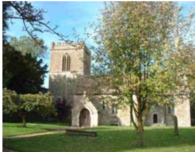
47 St John the Baptist's Church, Hinton Charterhouse
