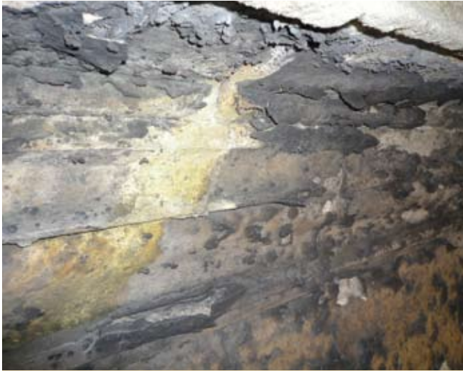
The surface of the stone starts to break up when the pores become blocked.
