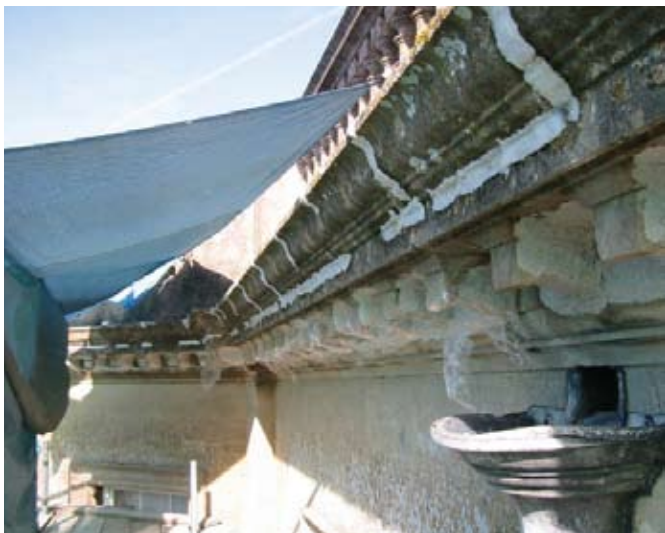
Poultices being used to remove specific soiling to this entablature.
