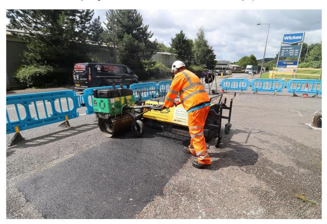
Benefiting from the proximity of a supplier just across the authority boundary in Somerset, we are now utilising a Viafix cold lay permanent pothole repair material supplied in bulk bags. The material typically is three to four times more expensive than traditional hot supplied asphalt concrete, but in bulk supply we have been able to agree a more agreeable cost.
