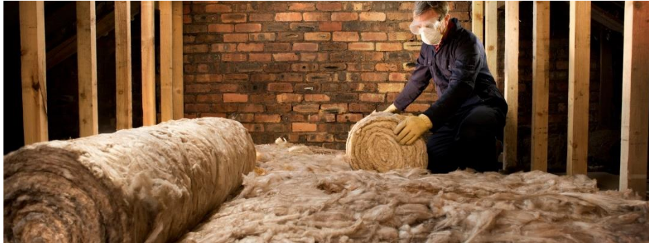
Pictured: A contractor installing loft insulation.
