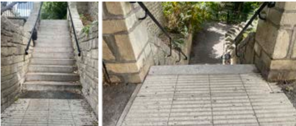
TACTILE PAVING AT THE TOP AND BOTTOM OF STEPS
