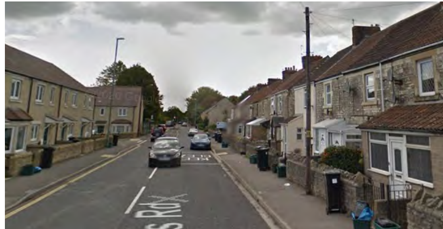
Example of a new development fronting onto the existing highway and is part of the streetscene. Taken from google streetview
