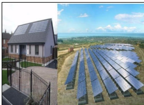
Figure 33: A Rooftop and Ground Mounted Solar Array
