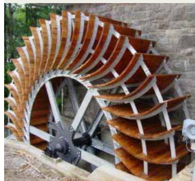
Bathampton Mill Hydro Scheme
