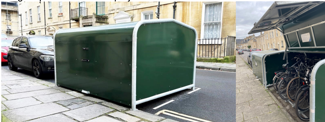
Figure 1 Existing cycle hangars in Bath
