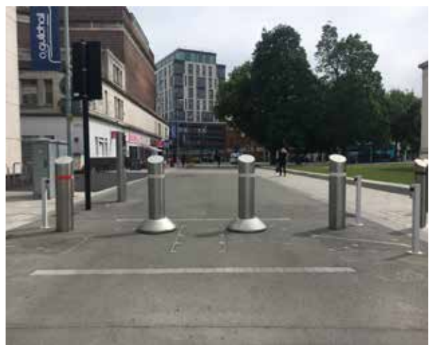
Moving bollards in Southampton
