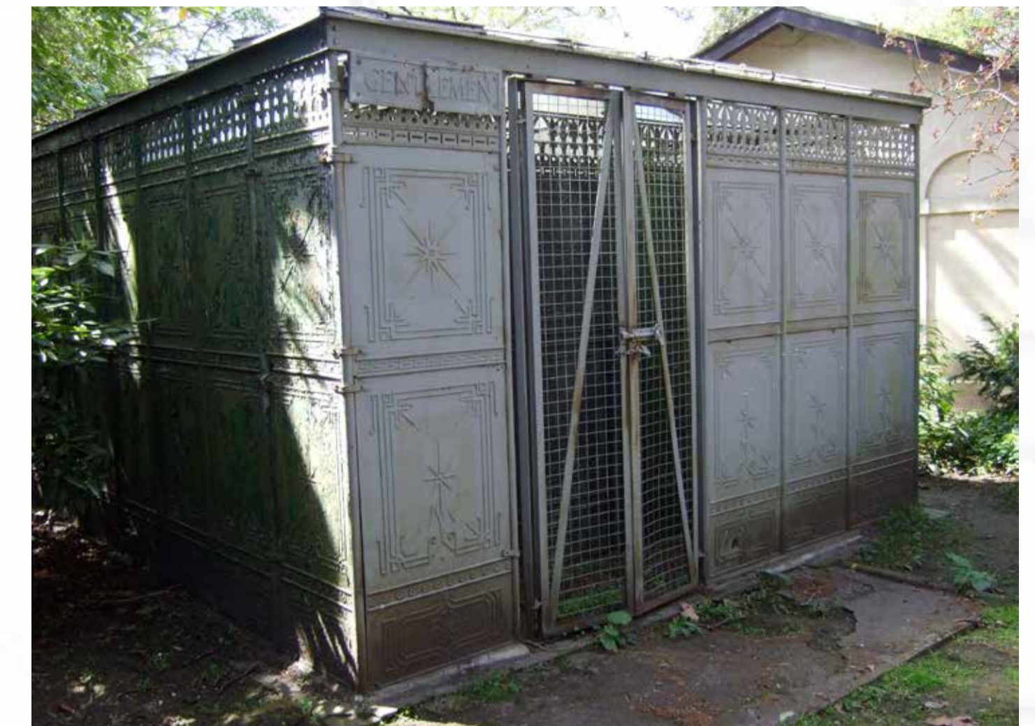
Cast iron toilet - Gentlemen Victorian toilet with ornate metal work and glass roof Proposal: Restore structure
