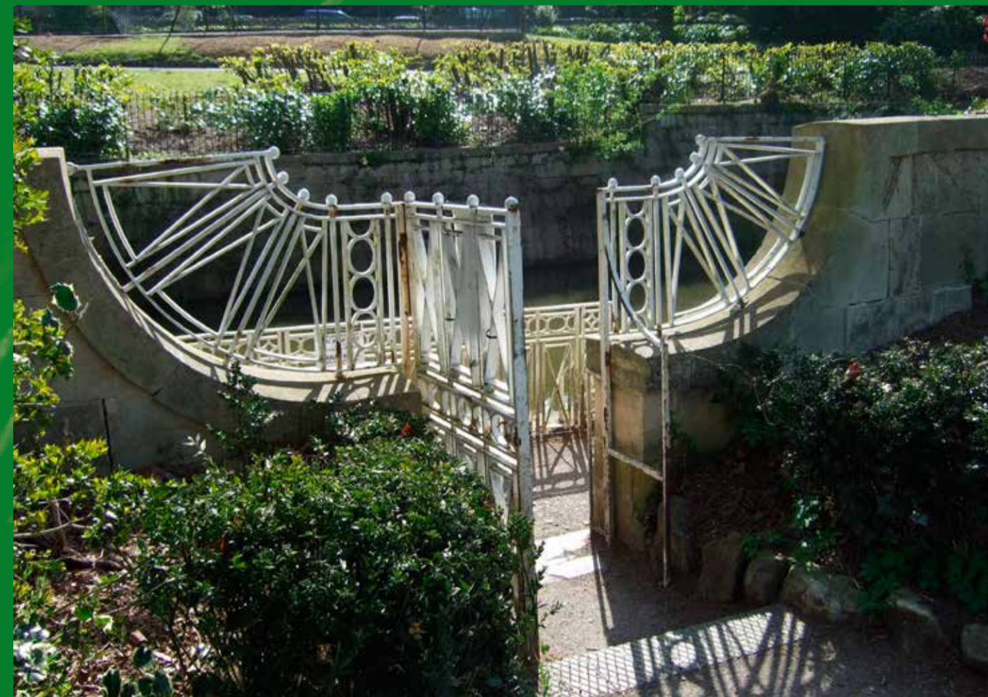
Access to towpath Only access to the towpath within the park creating a bottle neck. Proposal: Improvements to entrance and increase accessibility
