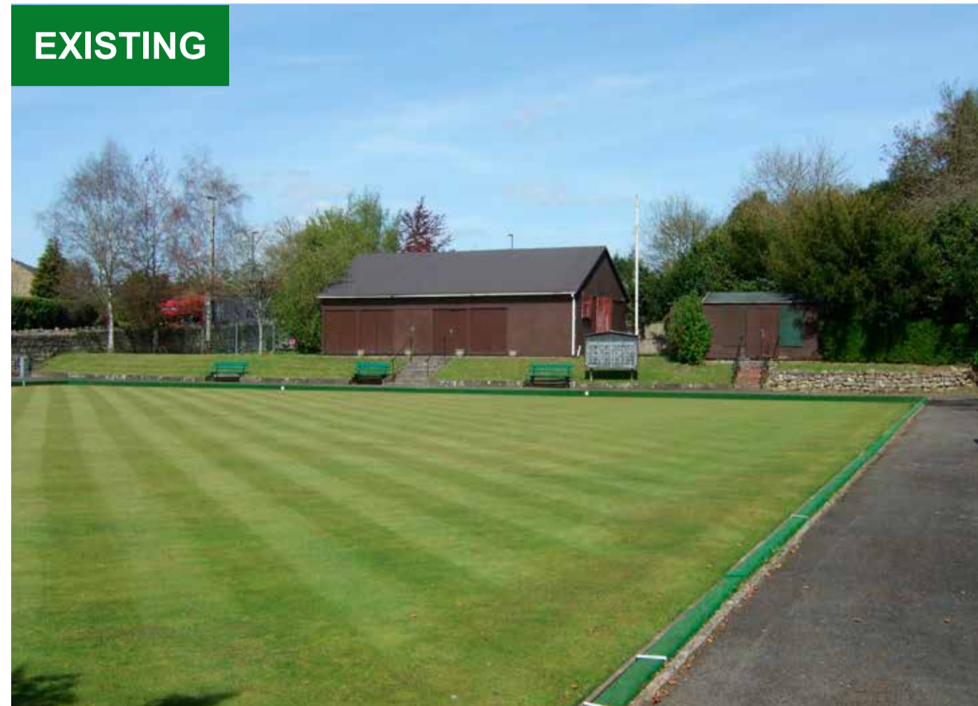
EXISTING Bowl's Pavilion Existing facility limited to use by Bowl's Club.
