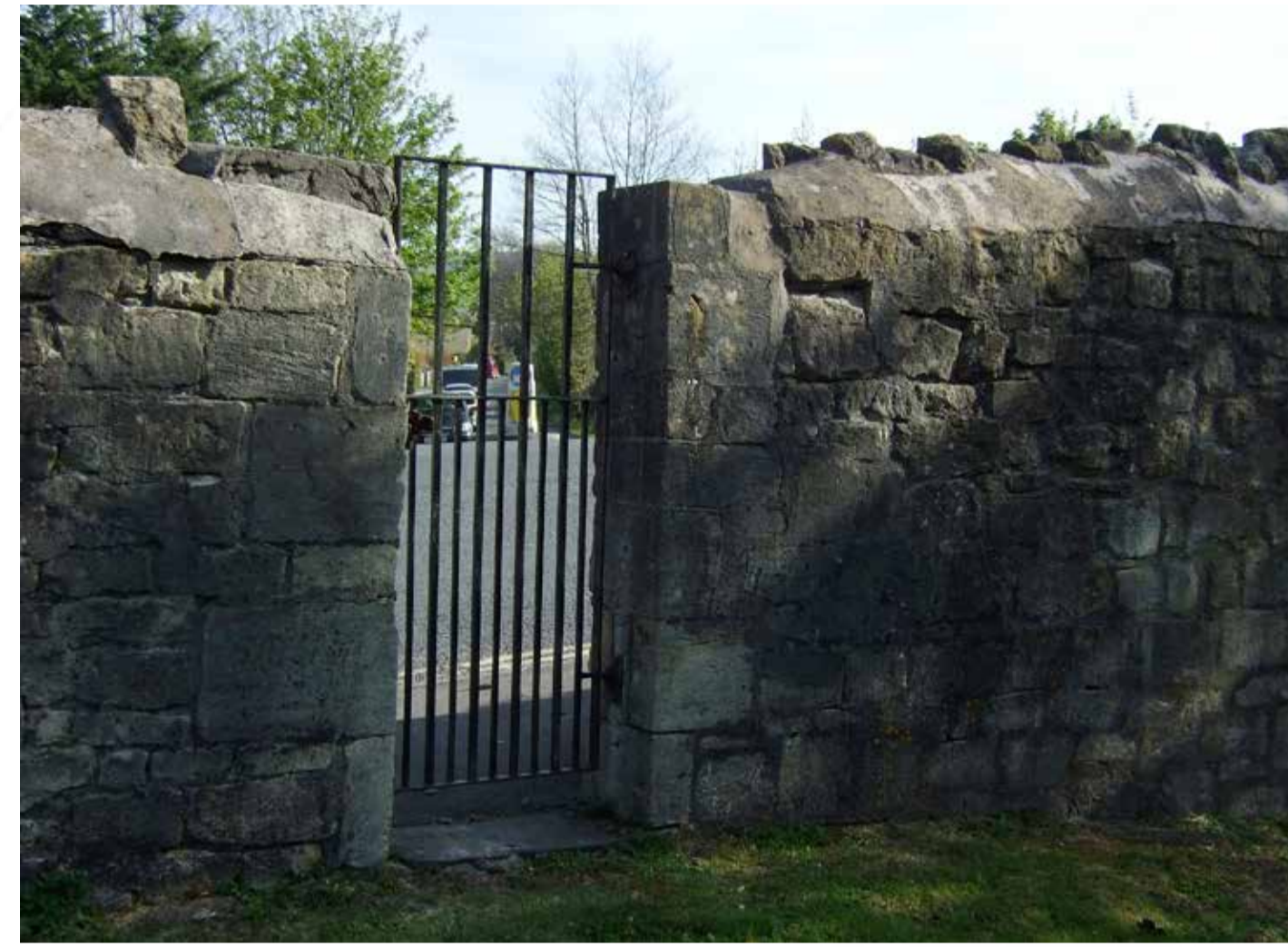
Gated access to Beckford Road Entrance is currently locked. No access to Beckford Road along this park boundary. Proposal: Reopen gate and provide a footpath connection into the park
