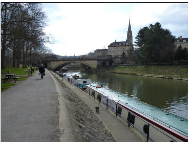
The Flood Alleviation Scheme through Bath
