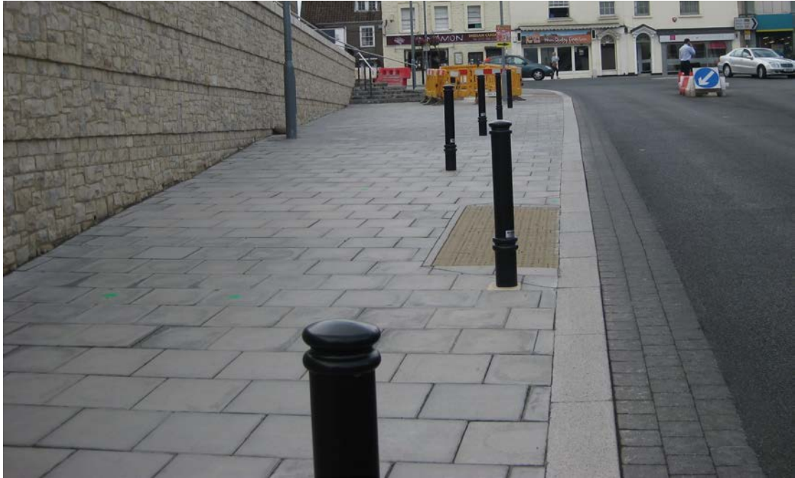
New pre-cast concrete paving slabs by the Town Hall with low height kerb and block channel. This paving layout could be extended along the High Street
