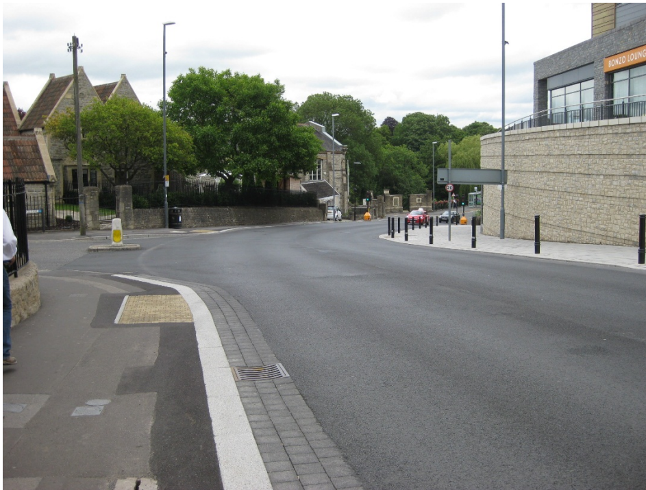
Recently completed scheme at Bath Road with low height kerbs and block channel. The road width is still relatively wide. Grey paving slabs are used on the footpath. The use of these materials can be extended into the High Street.
