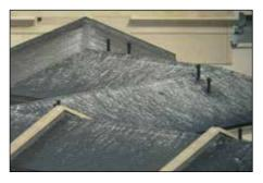
Wires can be stretched across a flat roof. These are aligned in parallel rows at a distance that will prevent a gull from landing. They have the advantage that other birds do not get snagged in them, and they can be less visually intrusive than nets.
