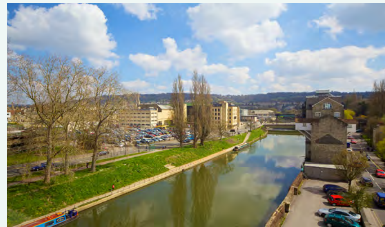
(below) Bath Quays today, showing engineered bank and flood walls
