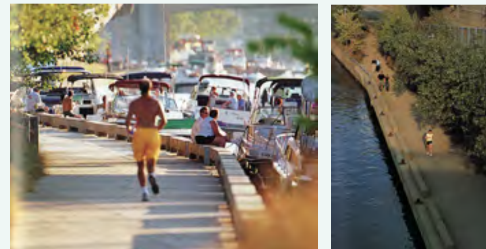
Pittsburgh has integrated flood protection engineering into a new waterfront alongside the river Allegheny, to create new moorings, a linear walkway, and plenty of greenery
