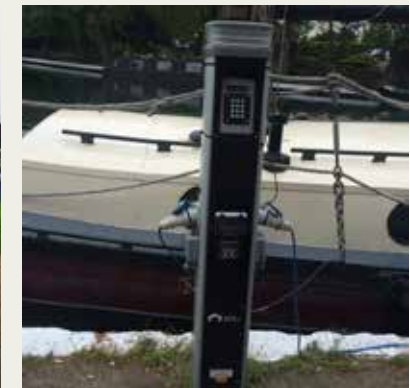
Electricity points to improve moorings and minimise the impact of generators and wood smoke
