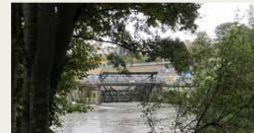
Twerton Water Level Control Gate
